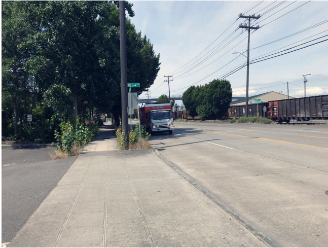
Figure 8 SW Idaho St BEFORE
