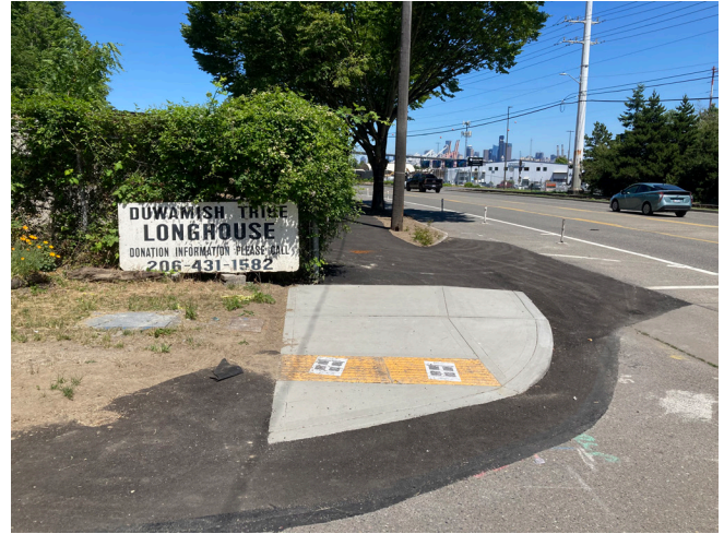
Figure 13 Duwamish Longhouse Walkway AFTER
