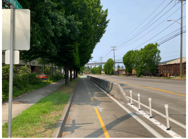
Figure 9 SW Idaho St AFTER
