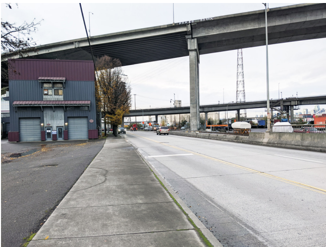
Figure 2 Southbound Lane Drop Under the West Seattle Bridge
