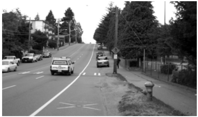
NE 130th St before lane reduction.
