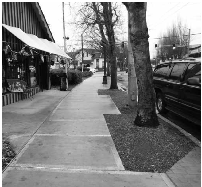
Sidewalk and drainage improvements along Rainier Ave S in Columbia City received funding from the NSF program.
