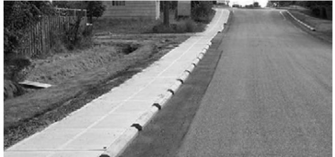
Curb-separated path at the same level as cars at N 97th Street and Fremont Avenue N.
