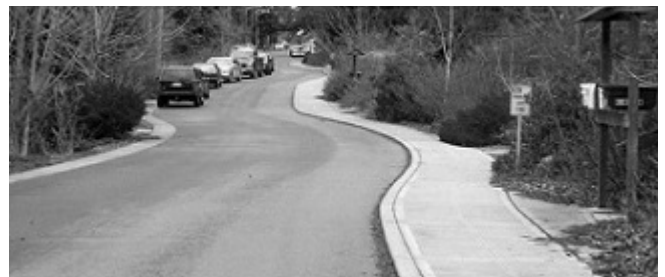
Conventional concrete sidewalk with curbs on one side of the street only, with bioretention that could be implemented in coordination with Seattle Public Utilities to keep costs low. 2nd Avenue NE pictured above.
