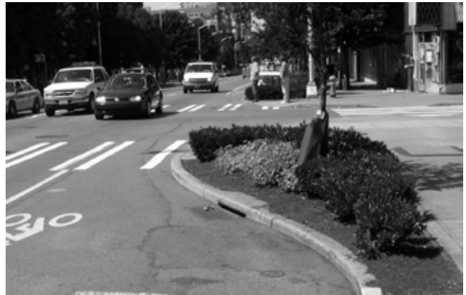
Curb bulbs in Belltown help narrow crossing distances for pedestrians crossing busy downtown arterials.
