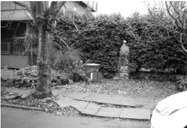
Tree roots can damage sidewalks and make travel difficult for pedestrians.
