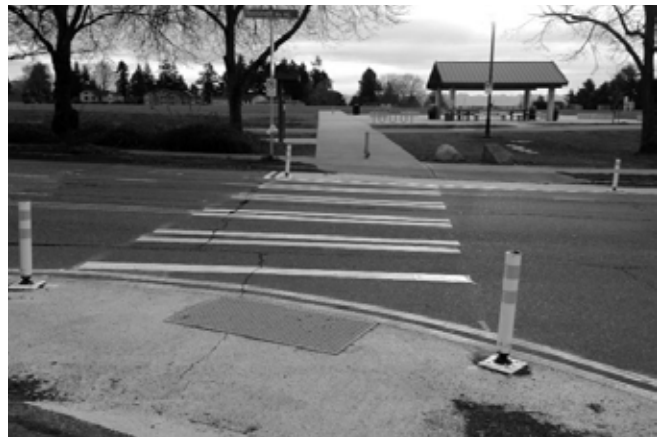
Painted curb bulbs in Maple Leaf, with safety pylons, help make pedestrians more visible and reduce crossing distances to Maple Leaf Park.
