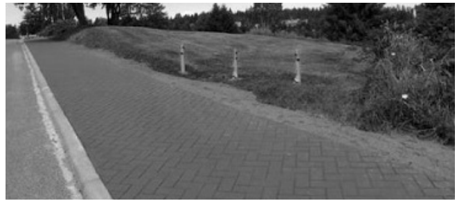
Stamped and stained asphalt sidewalk with curb (raised walkway) along NE 105th Street.
