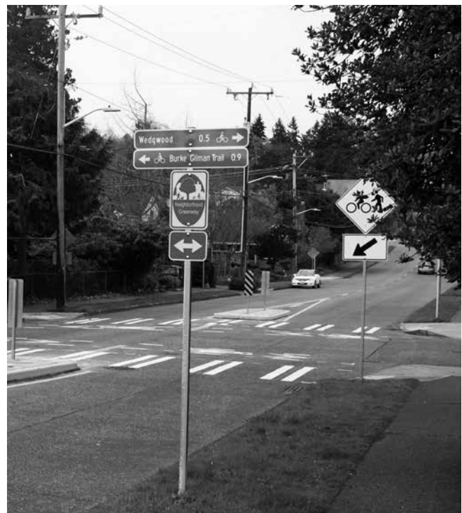
Improved crossing along the 39th Ave NE Neighborhood Greenway.
