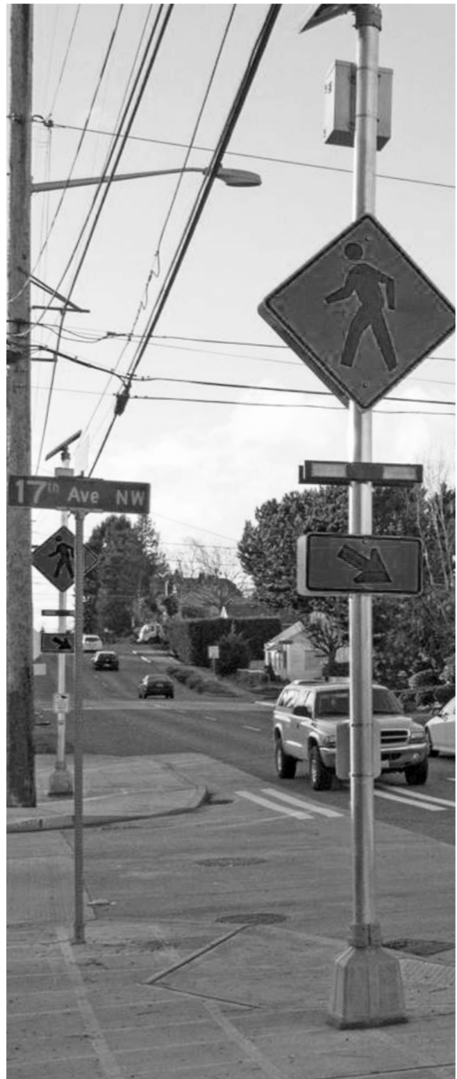
Crossing beacons, like this Rectangular Rapid Flashing Beacon (RRFB), have been shown to increase driver awareness of people crossing the street.
