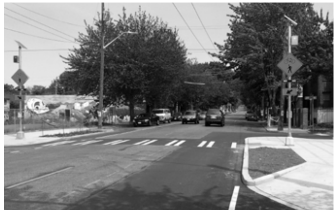
The Central District Neighborhood Greenway crossing at E Cherry St provides a crossing beacon to alert vehicles to people crossing the roadway.
