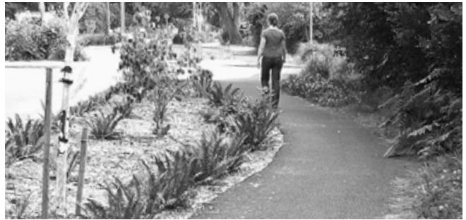
At-grade path behind green stormwater infrastructure without curb in the City of Shoreline.
