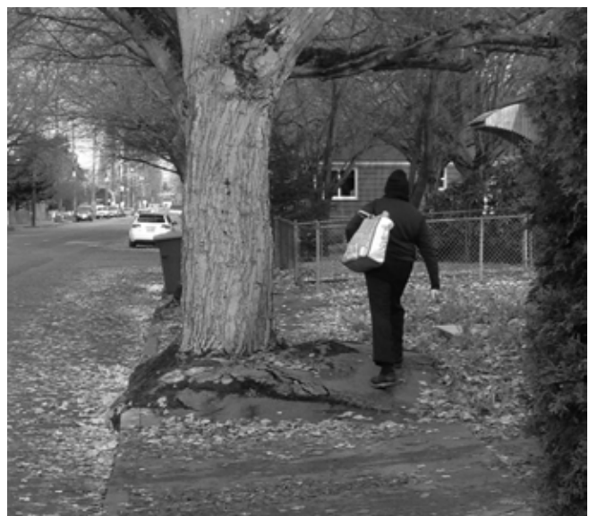
Tree roots can sometimes uplift sidewalks, making pedestrian paths difficult to navigate, especially for users with mobility challenges.
